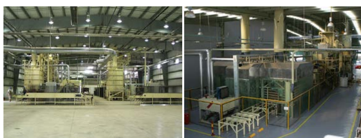
Figure 60. Compak line in Tongling, China
